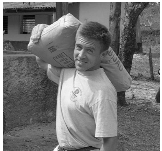
Bob Watson hauled lots of cement while working on the El Diviso water project in Honduras.
